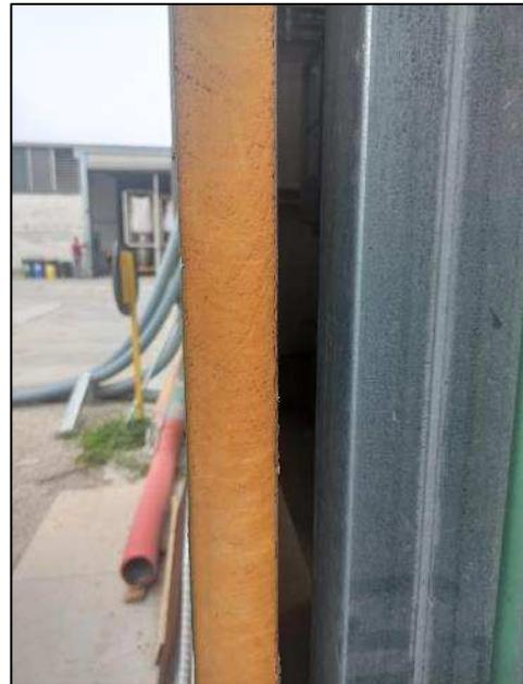
FIGURA 3-10 - DOCUMENTAZIONE FOTOGRAFICA ANTE OPERA (RIVESTIMENTO IN LAMIERA METALLICA) E POST OPERA (RIVESTIMENTO CON PANNELLO SANDWICH IN POLIURETANO SPESSORE 5 CM)
