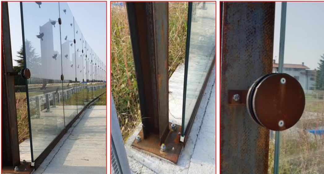
FIGURA 4-31. SCHEMA TIPO BARRIERA AUSTICA IN VETRO
